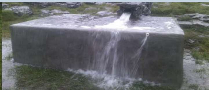
Clais éadomhain déanta timpeall ar an sruth amach as an tobar agus píopa curtha ann. Is féidir píopa a chur sa bpoll sa tanc le é a líonadh ón tobar. Shallow trough built around spring with out flow leading to bigger existing tank. Careful stone facing reduces the visual impact of the tank and the pipe work.
