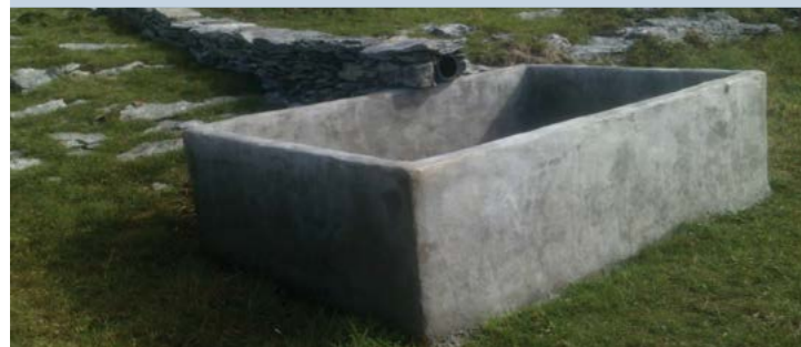
Clais éadomhain déanta timpeall ar an sruth amach as an tobar agus píopa curtha ann. Is féidir píopa a chur sa bpoll sa tanc le é a líonadh ón tobar. Shallow trough built around spring with out flow leading to bigger existing tank. Careful stone facing reduces the visual impact of the tank and the pipe work.
