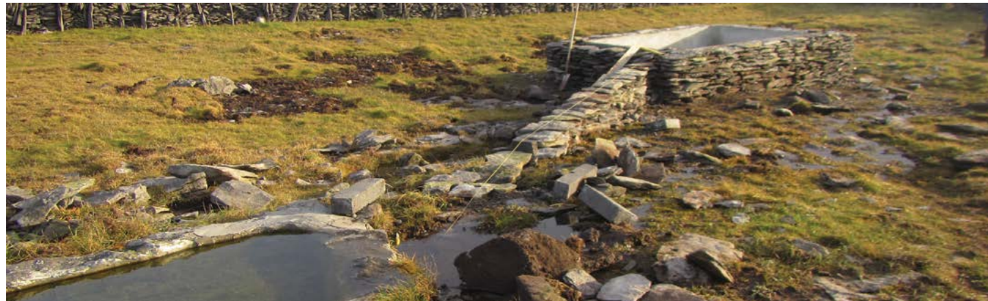
Clais éadomhain déanta timpeall ar an sruth amach as an tobar agus píopa curtha ann. Is féidir píopa a chur sa bpoll sa tanc le é a líonadh ón tobar. Shallow trough built around spring with out flow leading to bigger existing tank. Careful stone facing reduces the visual impact of the tank and the pipe work.
