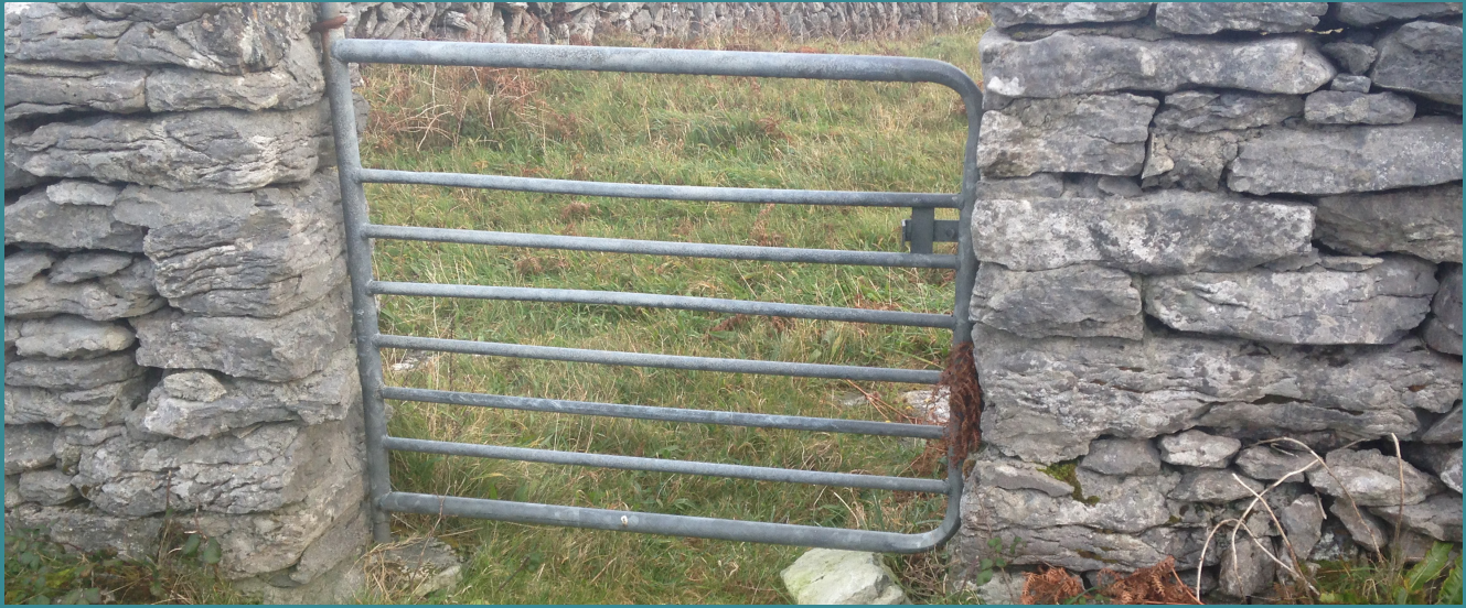
Sampla de gheata ar bhuaile agus taobhanna an chlaí á n-úsáid mar phostáí. An example of a field gate using incorporating the pillars into the existing stone walls.
