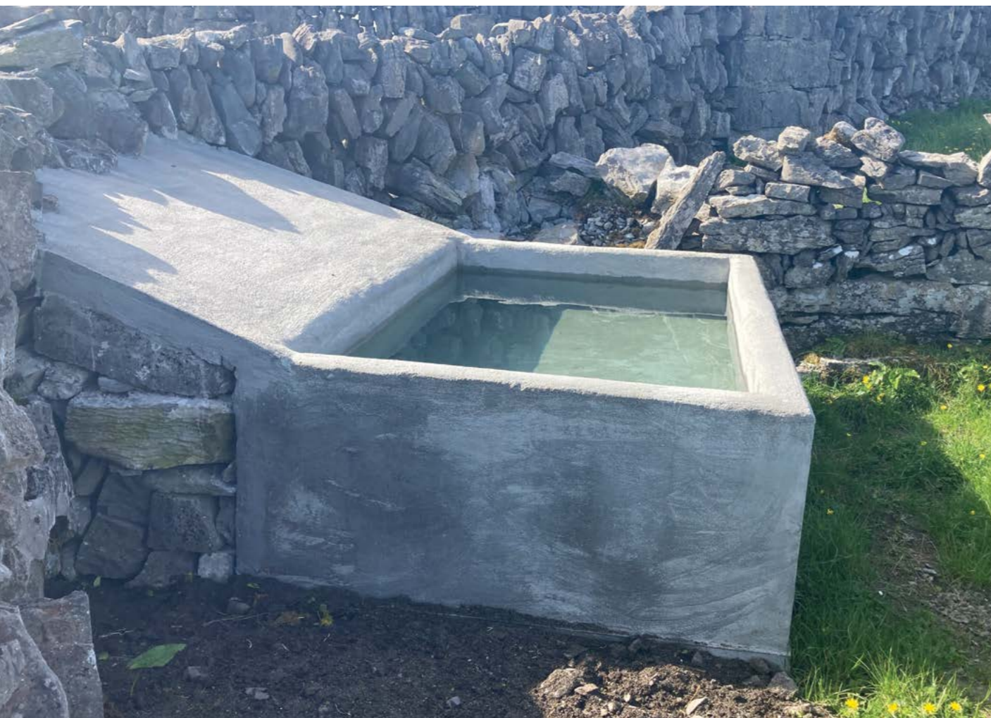
Fig.13 Construction of traditional raincatcher
